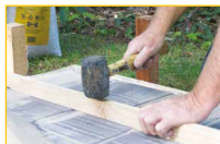
Tamp sand into paver gaps
