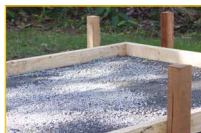
Prepare road base
