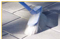
Broom sand into gaps
