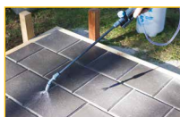
Thoroughly wet paving
